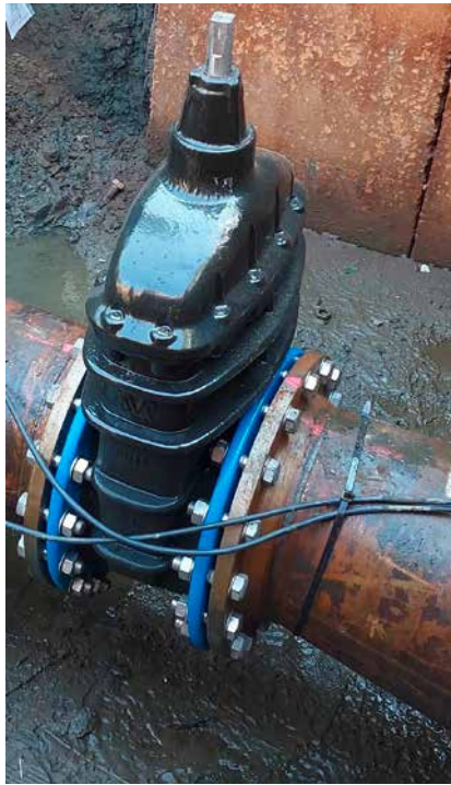
An AVK PREMIUM100 gate valve installed in the system, and one of the old, now replaced valves.
